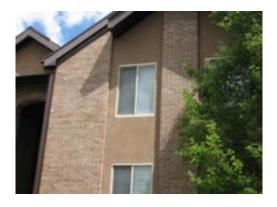
Stucco appears to be newer and in good condition. The stucco has embedded color and should last a long time however once repainted it will need to be painted every 8 years.
